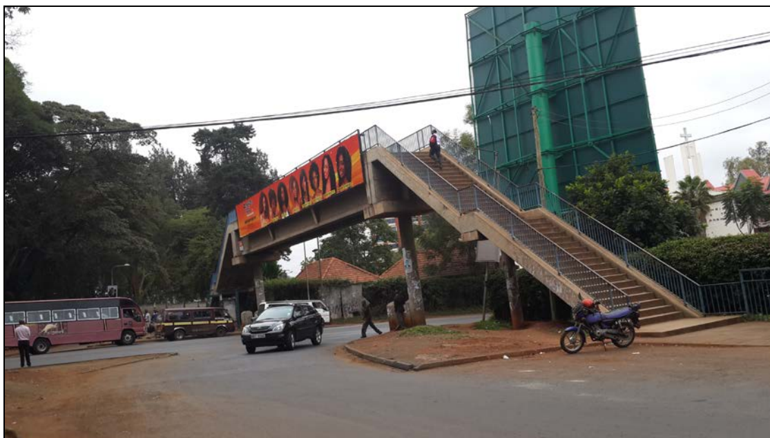
Plate 5.8: A foot bridge over valley road
