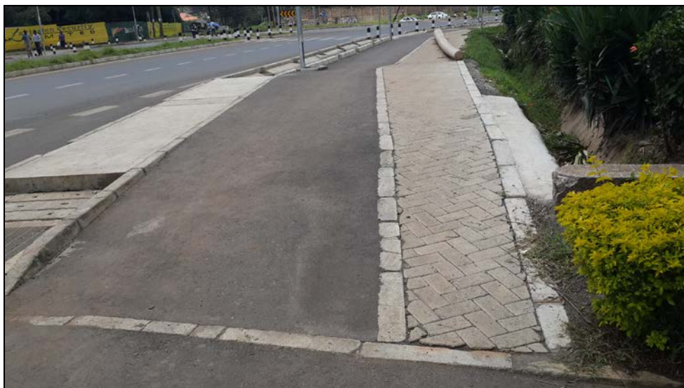
Plate 5.2: A section of the Kilimani Ring Road footpath accessible by PWDS on wheelchair
